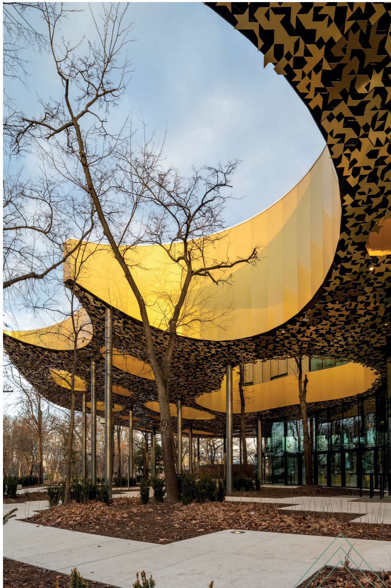
House of Music, Hongrie | Sou Fujimoto Architects | ALUCOBOND® PLUS spectra Desert Gold | © György Palkó
